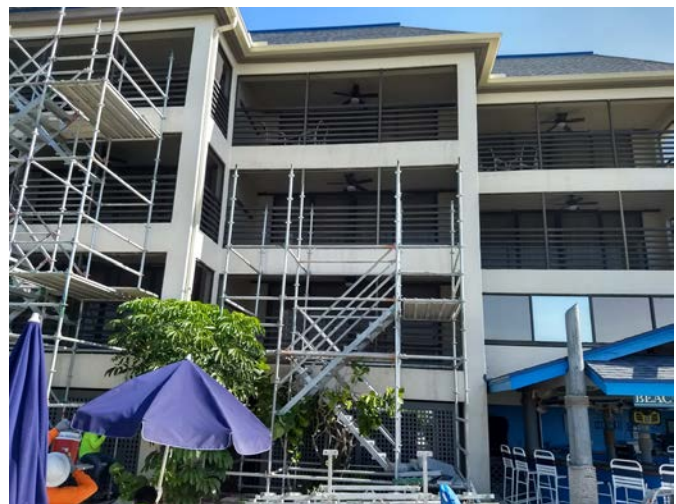
Scaffolding erection at lanai stack 6.
