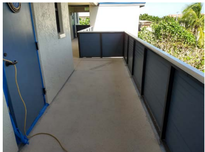
Walkway at Unit 306 – old floor coating removed.
